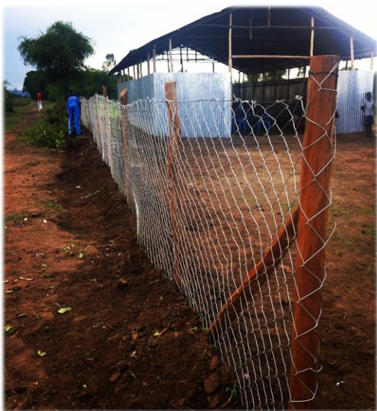
Church in the background with the new fence.
