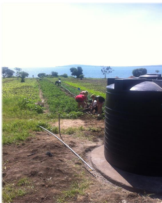
Attaching the new pipes for irrigation together with some local plumbers.
